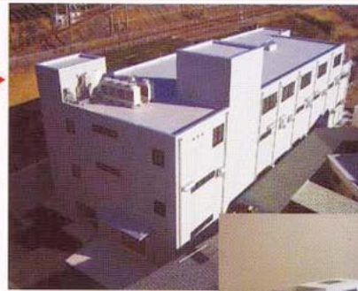
新商品開発工場 New Building to Develop New Product
